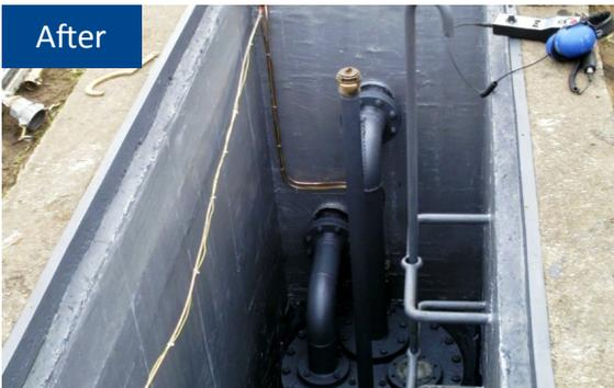
Using specifically designed and certified composite materials, the sump becomes a liquid-tight container to protect the floor from contamination. The coating also reinforces the sump's structure and protects the metal parts against corrosion.
