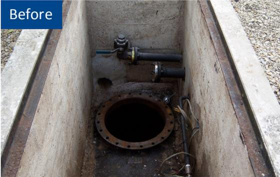
Sumps are a critical element of all storage facilities for potential contaminating liquids. This is especially important during the product transfer where the liquids can get in contact with the walls of the sump. Our sump refurbishing systems makes these surfaces liquid-resistant again.
